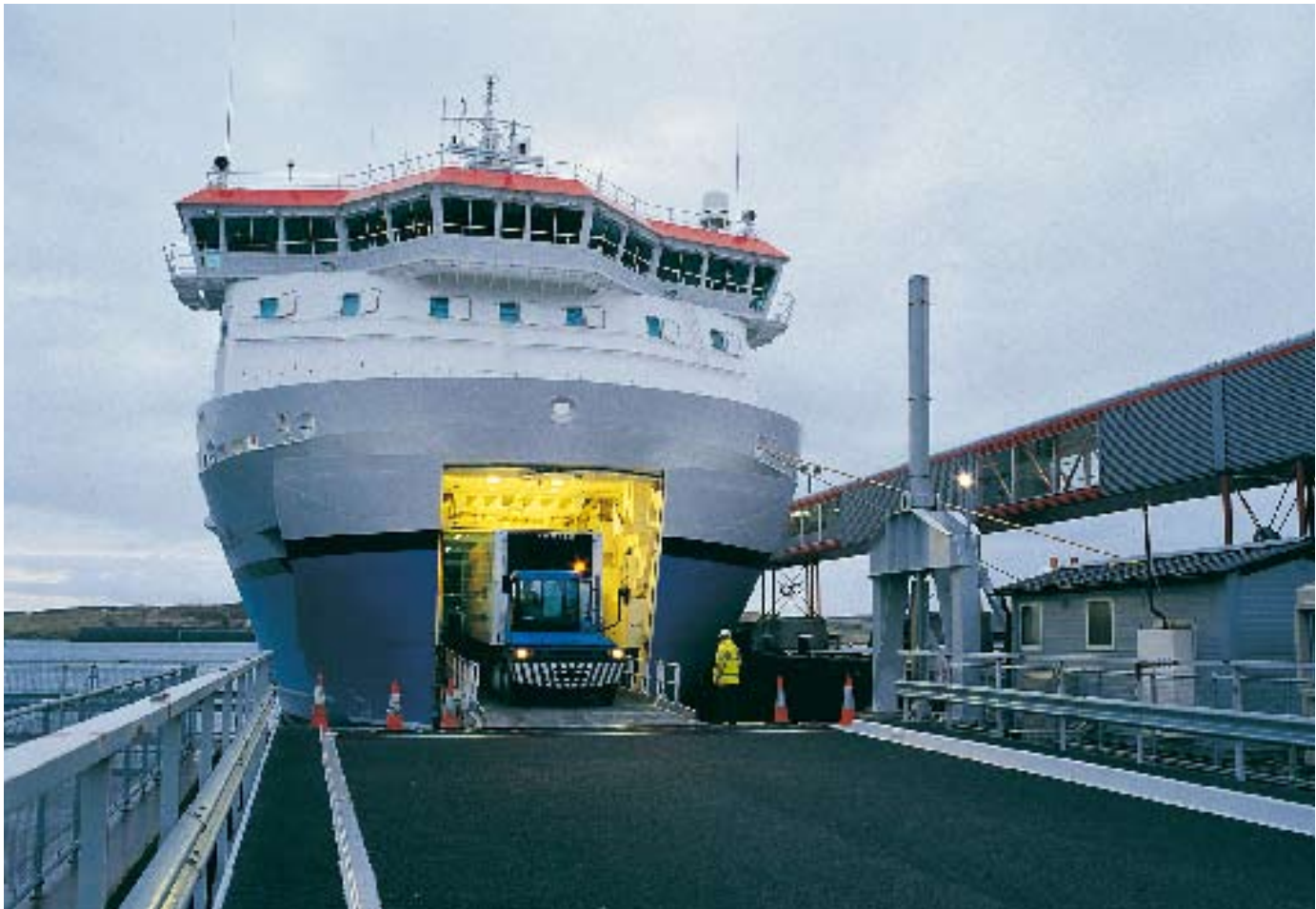
HJALTLAND at Lerwick, showing the new link-span and the airport-style enclosed boarding bridge at the right.
